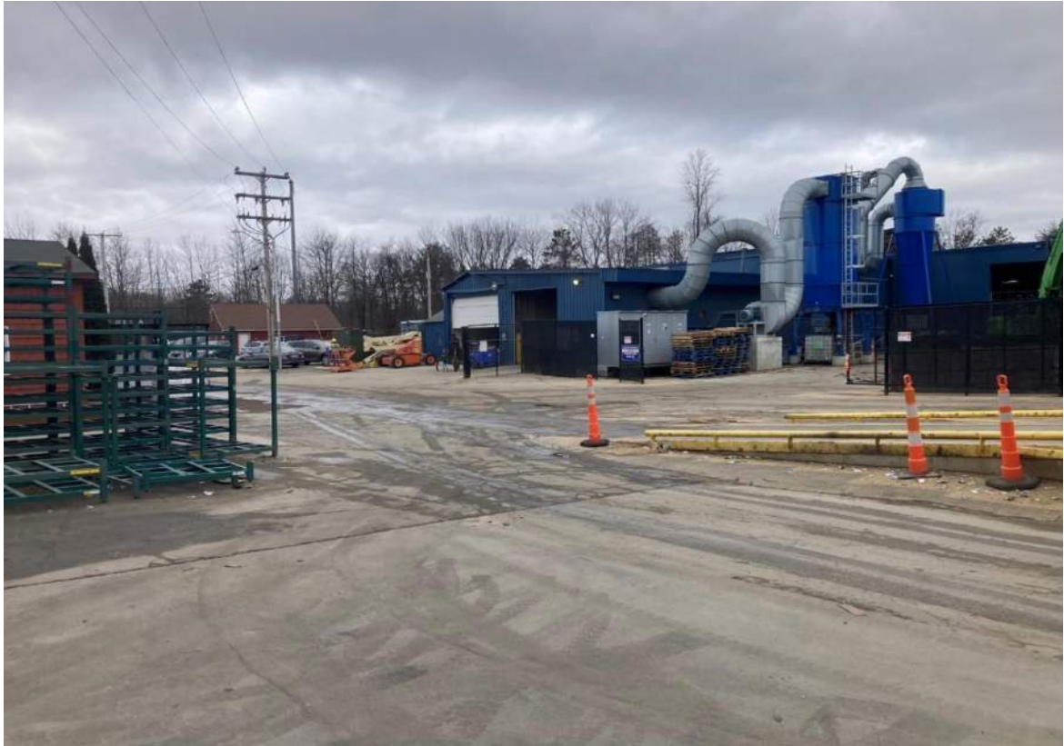
Photo 3: One-story metal frame building, facing West.
