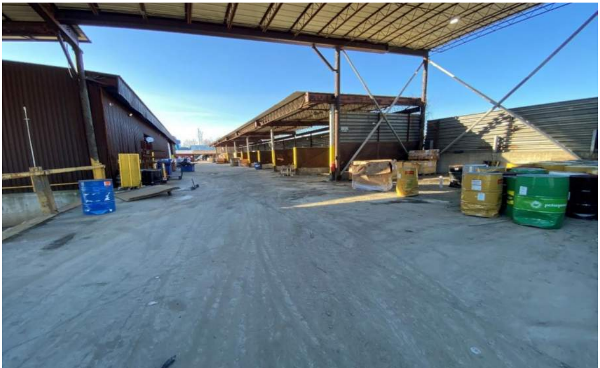
Photo 8: Northern covered storage area and Two-story metal frame building, facing West.
