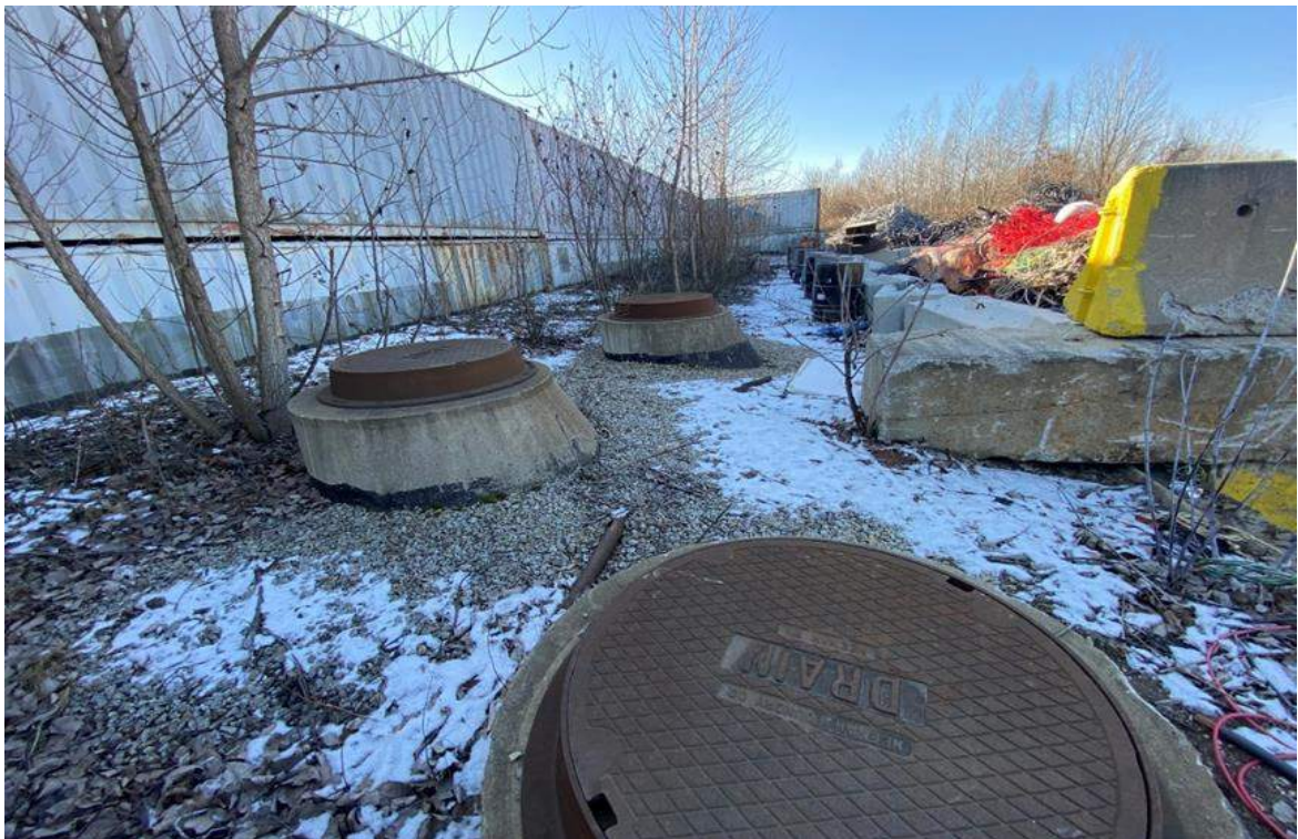
Photo 4: Approximate location of existing subsurface stormwater system, facing Northeast.
