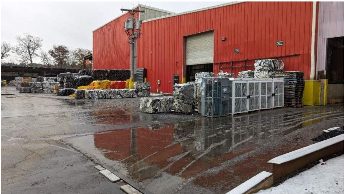
Photo 2: Two-story metal frame building, facing West.
